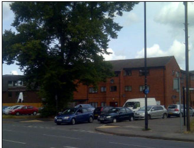
Image 2: South facing units in Kingsmead House
